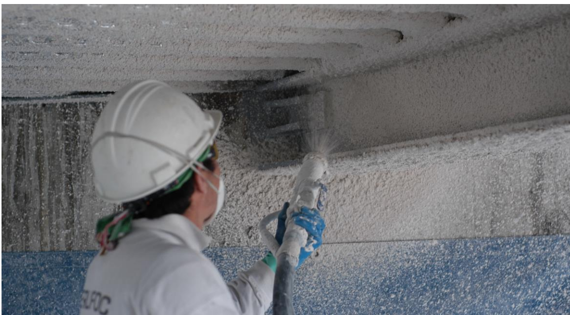
Picture 10 (Mortar spraying detail)
