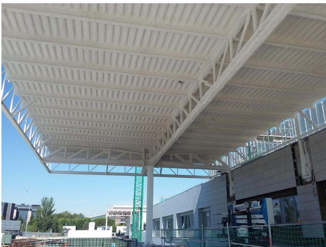
Picture 1 (Sprayed mortar on industrial warehouse)
