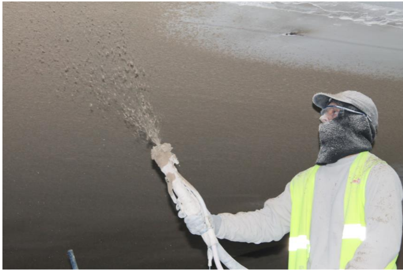
Picture 9 (mortar spraying application)
