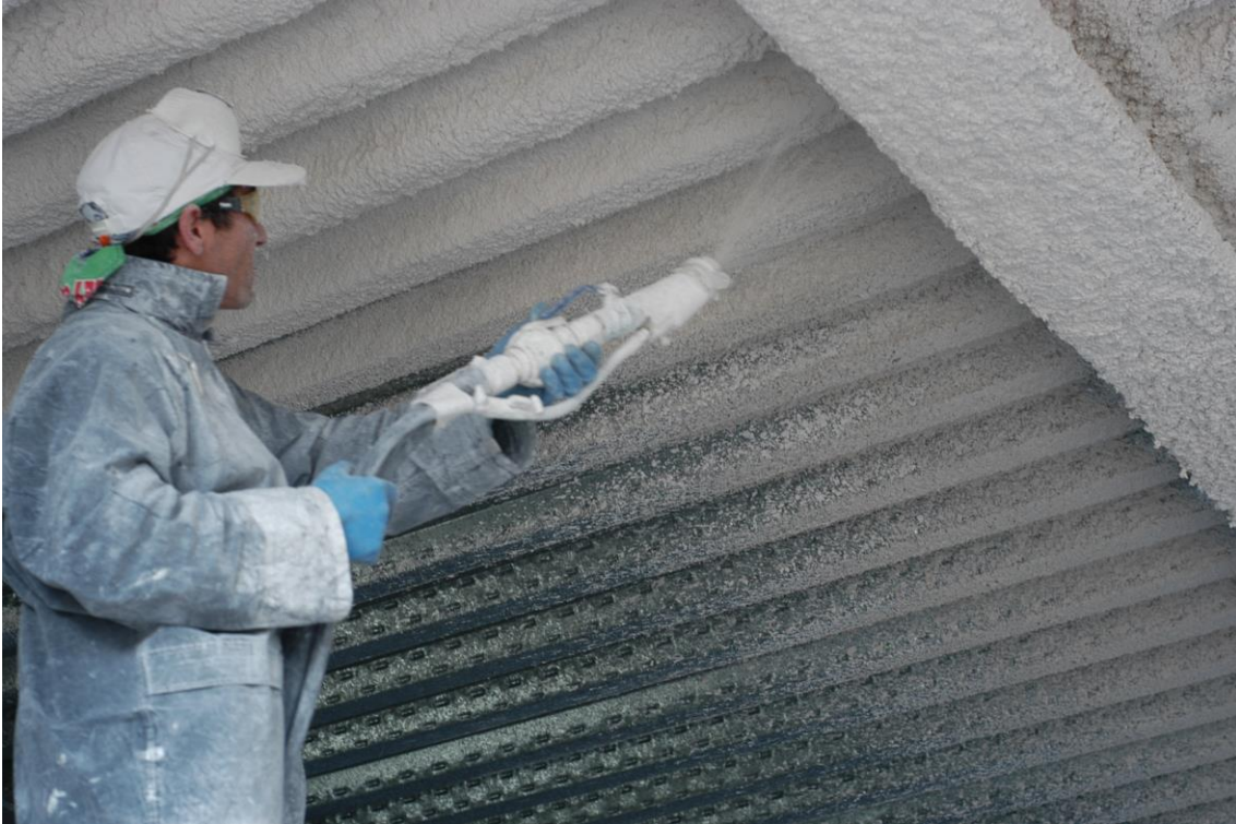
Picture 9 (mortar spraying application)
